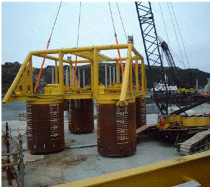
Figure 4.4.b. Subsea template at Kristin Field. (Nergaard, 2008)
